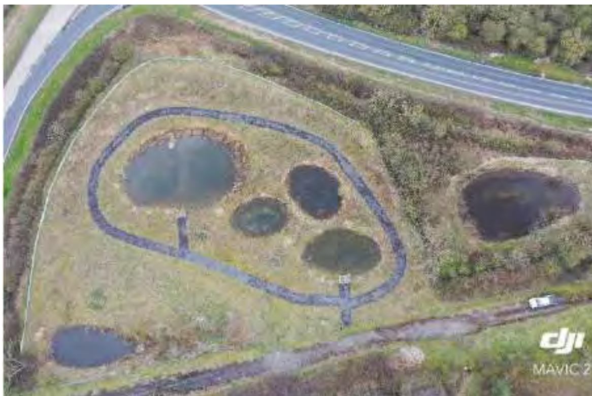
Figure 1-4: Mitigation Area B, Completed 2014
